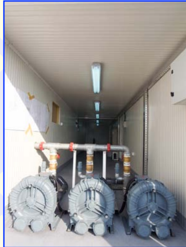
Side Channel Air Blowers. Efficient and quiet
